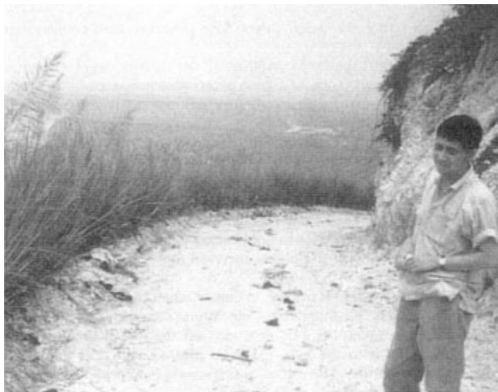
Vetiver stabilizing the edge of a hillside road, a common location for severe erosion. (P. Boyer)
