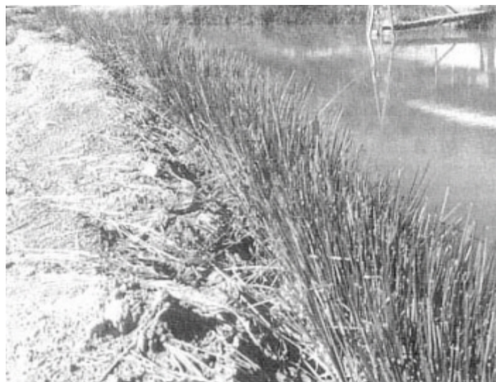
Vetiver hedgerows protecting newly formed embankments around a deep pond. This plant, which withstands wet conditions and even total immersion, seems an excellent candidate for protecting the edges of waterways of all types. (P.K. Yoon)
